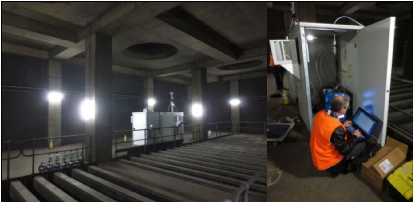
Figure 1. Installing measurement equipment in the CLEM7 Northbound tunnel vent.
