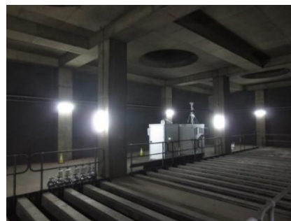
Figure 3. CLEM7 tunnel measurements in Brisbane.
